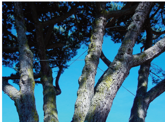
The limbs of this Stone Pine have been cabled together to reduce chance of failure.
