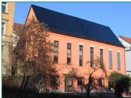
Roof-Mounted Photovoltaic CIS-Solar Cells photo by Björn Appel/Warden used via Creative Commons License
