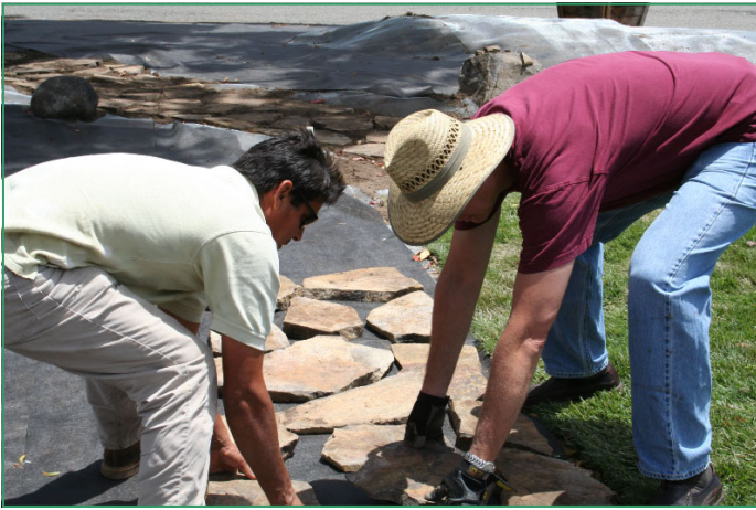
Baltazar Gutierrez and Greg Clinton lay stone paths in preparation for planting day.
