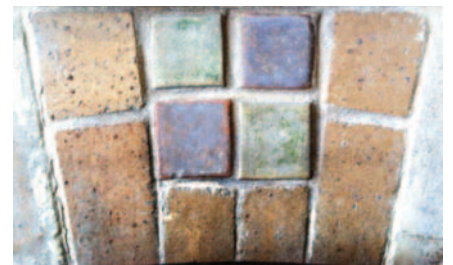
Glazed field tiles combined with sandstone brick —after paint removed
